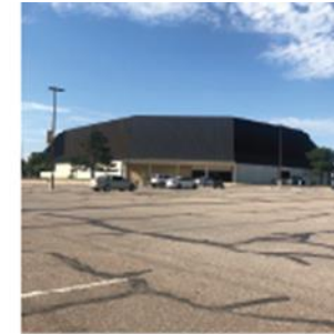
Gross Coliseum Roof Replacement R&R Funding
