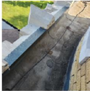
Albertson Hall Upper Level Roof Repairs R&R Funding
