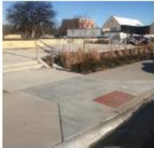
Sidewalk Repairs/Replacement General Repairs R&R Funding
