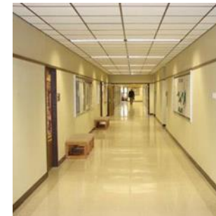
Rarick Hall University and Rehabilitation & Repair Funding Renovate and repurpose vacated space
