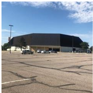
Gross Coliseum Rehabilitation & Repair Funding Roof Replacement
